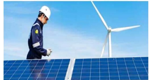
Installation of Renewable Energy Products and Systems
